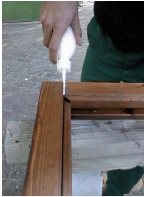
Fig. 7: application of the XA 481 single-component filler on the ends. First use the special doser to apply the product on the end section, then remove any excess product with your finger.
